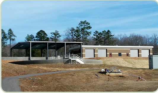
New Sludge Maintenance Building
